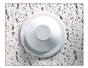
The Model F1FR-300 automatic sprinkler utilizes a 3.0mm frangible glass bulb. This sprinkler has demonstrated response times in laboratory tests which are five times faster than standard responses sprinklers. This quick response enables the Model F1FR-300 sprinkler to apply water to a fire sooner than standard sprinklers of the same temperature rating.
